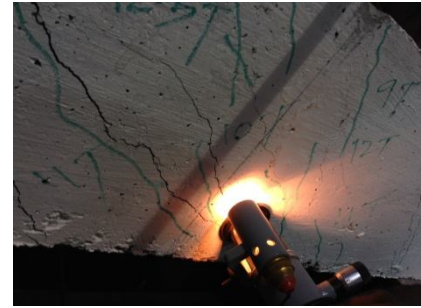
Figure 9. Measurement of Crack Width
