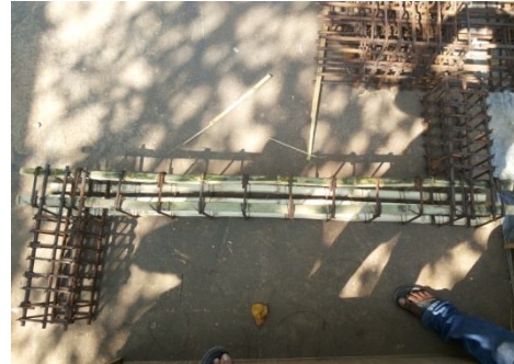
Figure 3. Prepared Reinforcement with Bamboo
